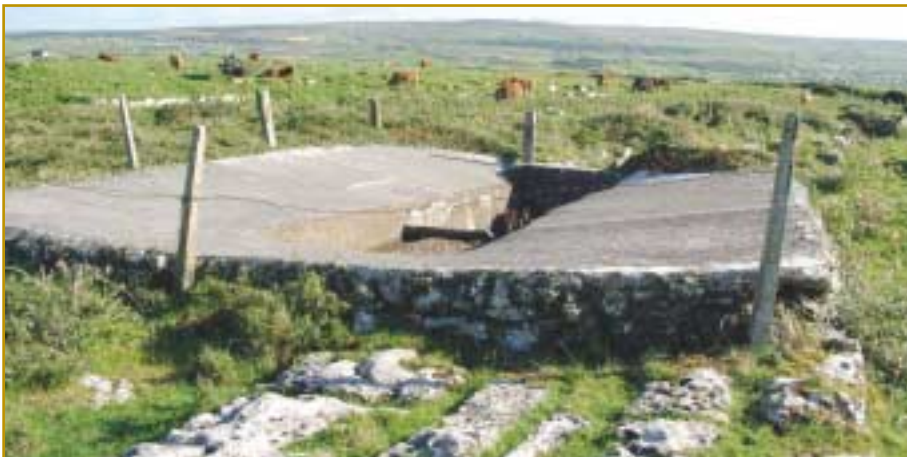
Rainwater collection and storage tank. The size, number and distribution of these tanks in the Burren uplands reflects the scarcity, and value, of a consistent water supply, a situation typical of karst landscapes all over the world.
