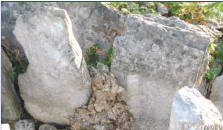
Scrub growth resulting in the severe disturbance of a court tomb structure.
